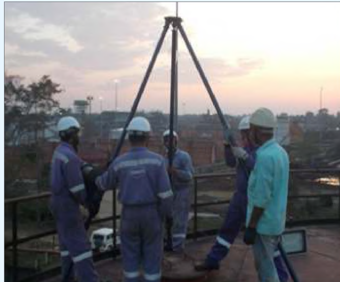
Photo 2: Support Erection for launch of rover
