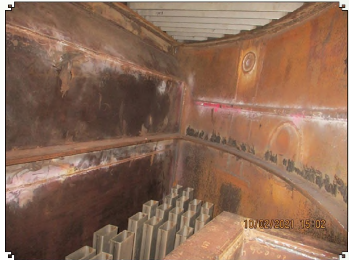
Figure 3: New Dividing Wall inside Splitter II
