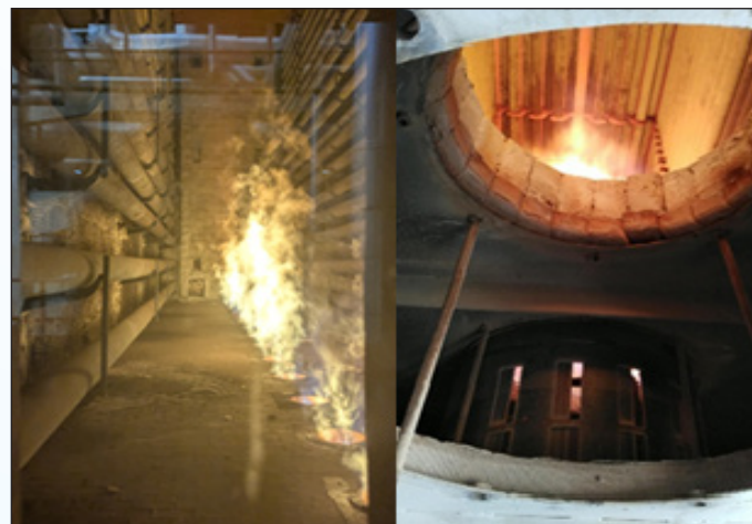
Figure 1: Stable flame vs. Impinging Flame
